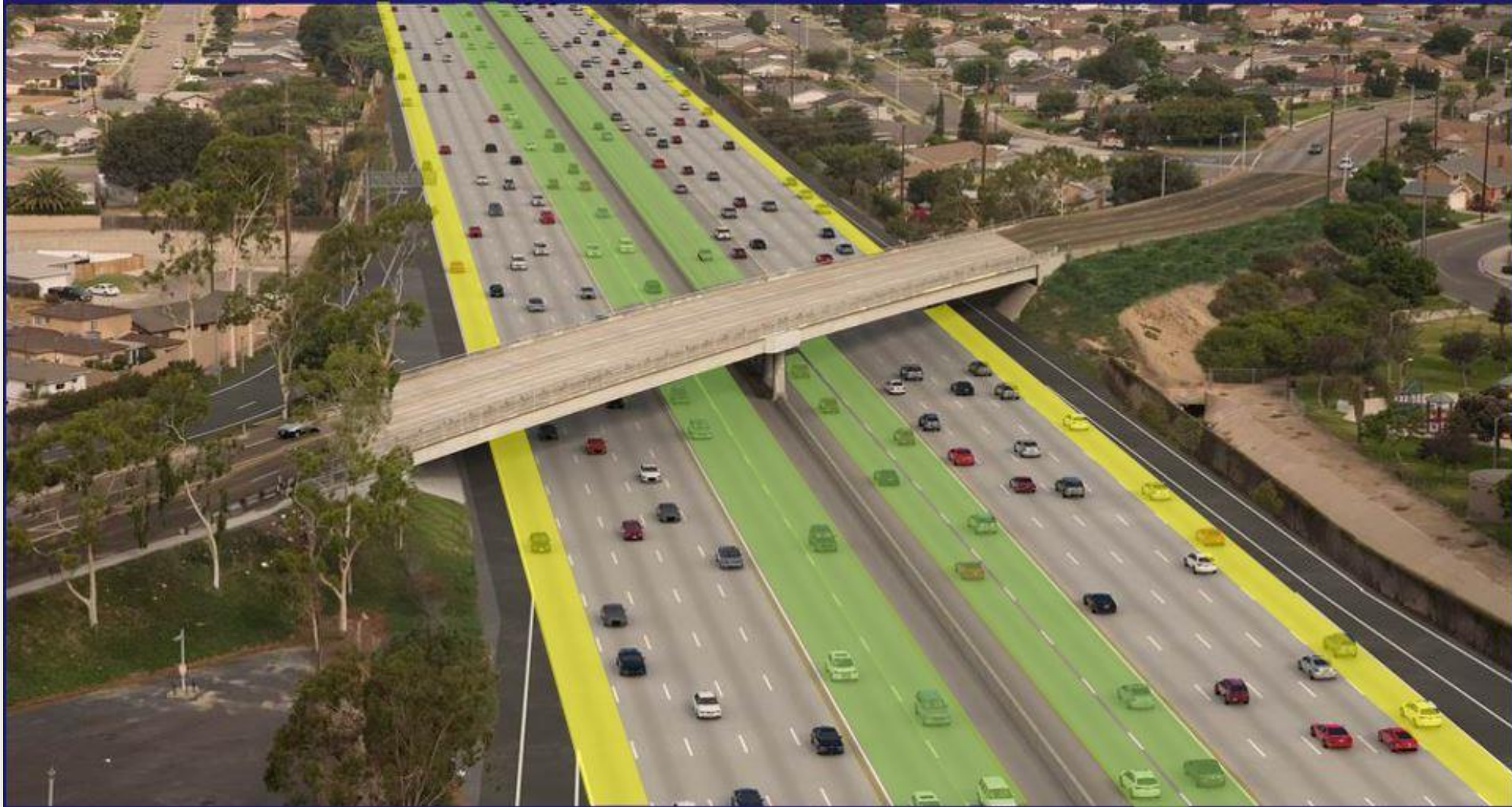
I-405 looking northwest at Springdale Street bridge
